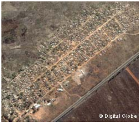
Before the destruction of Porta Farm, Zimbabwe (22nd June 2002)
